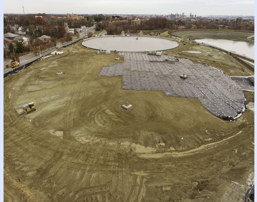
Installation of Geomembrane on top of Tank A & Backfill of Tank B – 11/27/2024
