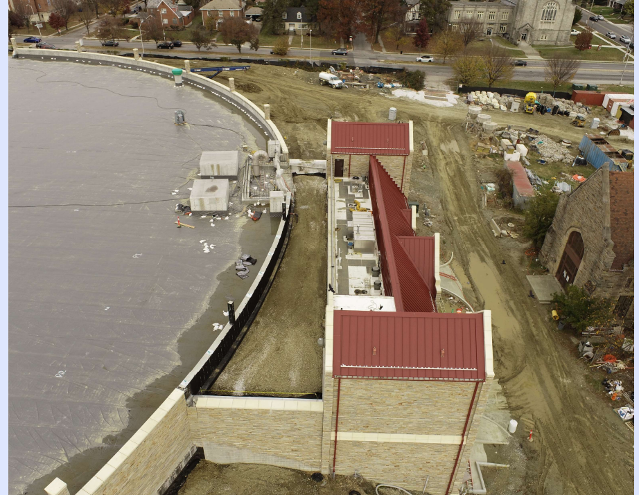
Backfill of Wing Walls – 11/27/2024
