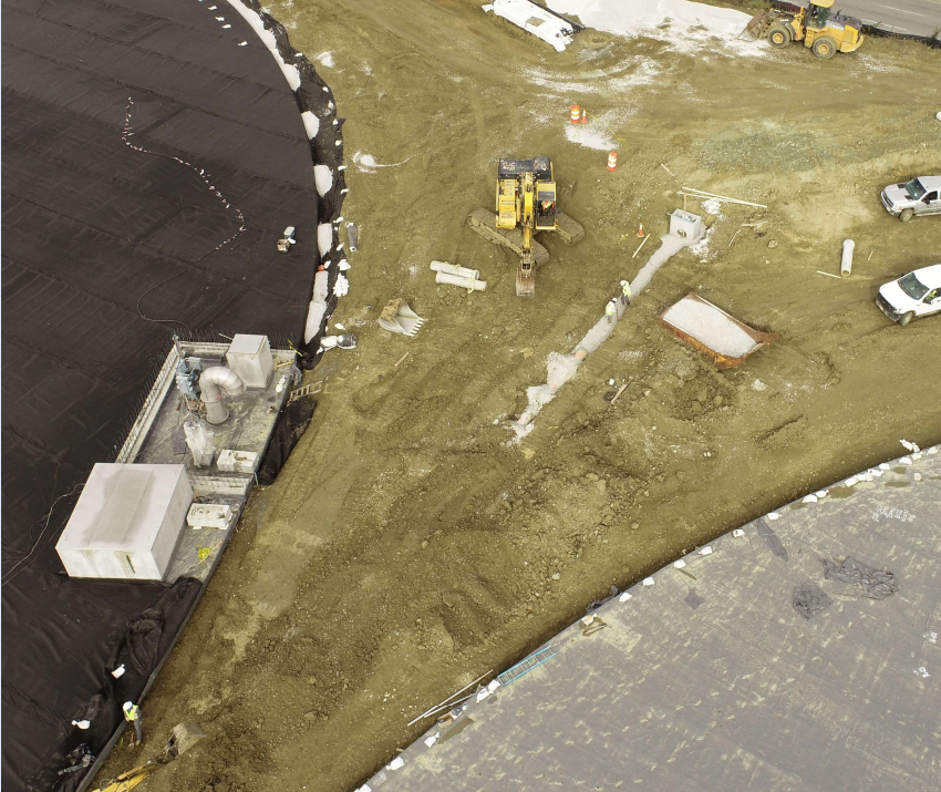
Storm Water Piping Installation – 11/15/2024
